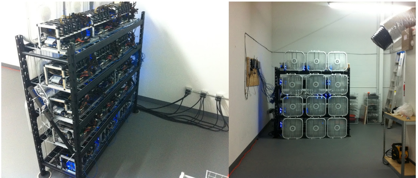
Figure 5: Two pictures of a homebrew 69-GPU Bitcoin mining data center. Note the ample power delivery on the photos on the left, and the cooling system, consisting of the box fans and air duct on the photos on the right. The GPUs are arranged in racks as shown in Figure 4. Photos Credit: James Gibson (gigavps).
